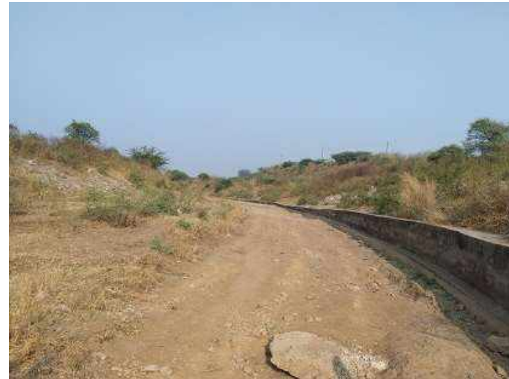
IMAGE-6 DIVERTED KORADI NALA AND STONE PITCHING ALONG WITH RETAINING WALL (Source: WCL)
