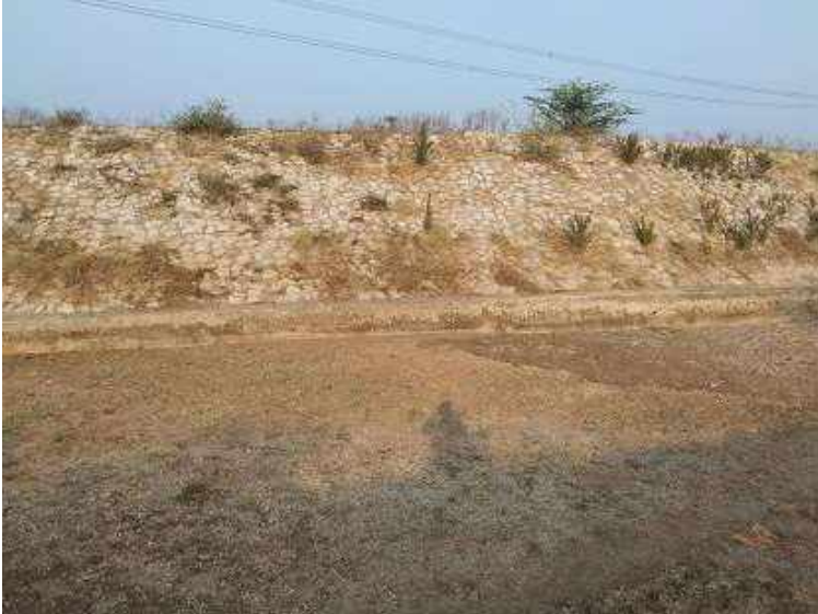
IMAGE-6 DIVERTED KORADI NALA AND STONE PITCHING ALONG WITH RETAINING WALL (Source: WCL)
