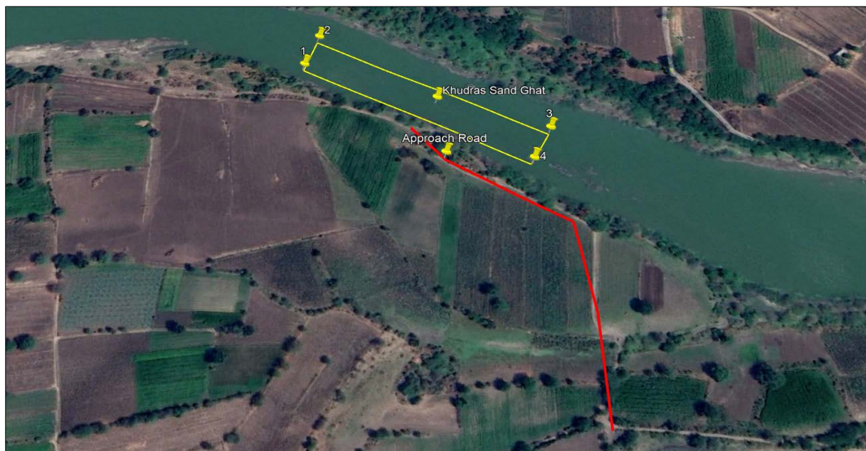
Fig 2.2-Approach Road for sand ghat
