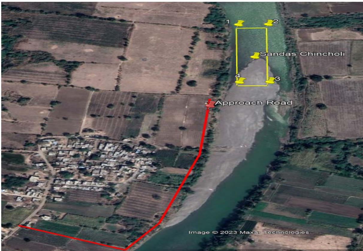
Fig 2.2-Approach Road for sand ghat
