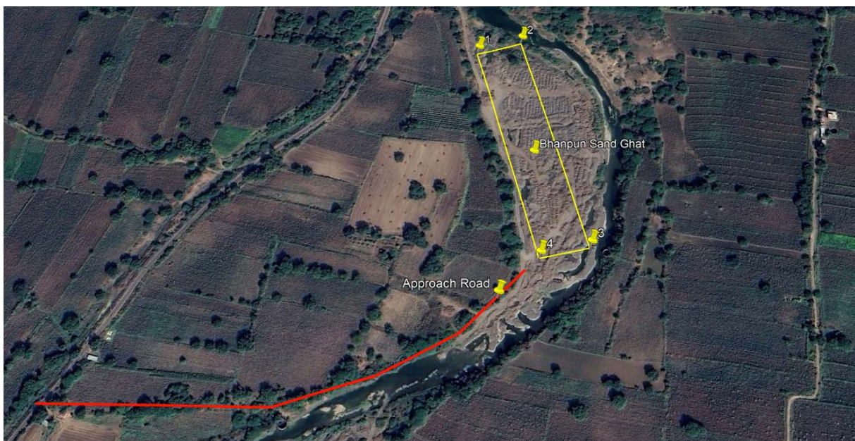
Fig 2.2-Approach Road for sand ghat
