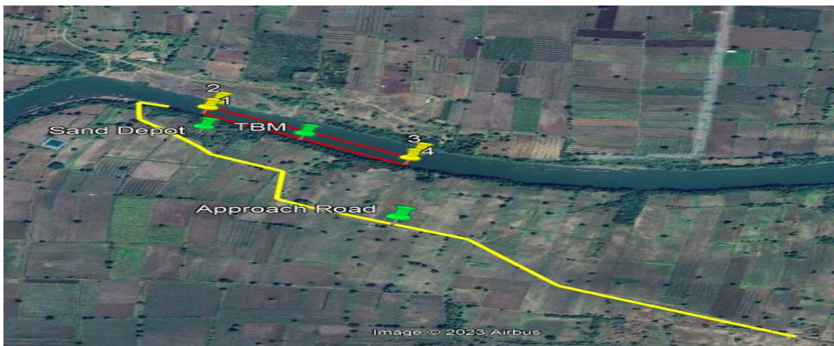
Fig 2.2-Approach Road for sand ghat
