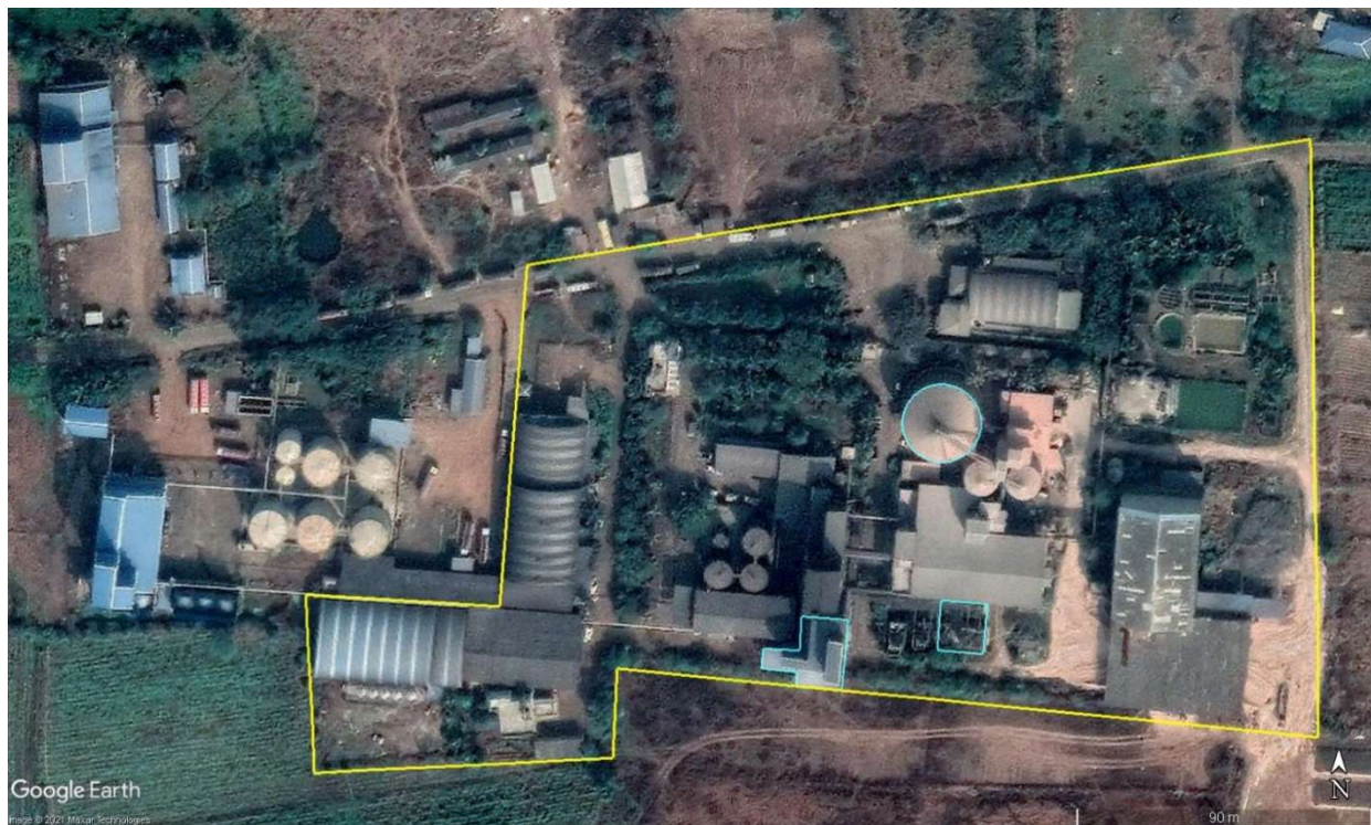
Figure 8 VAAIL Premises with Additional Infrastructure Created on Site
