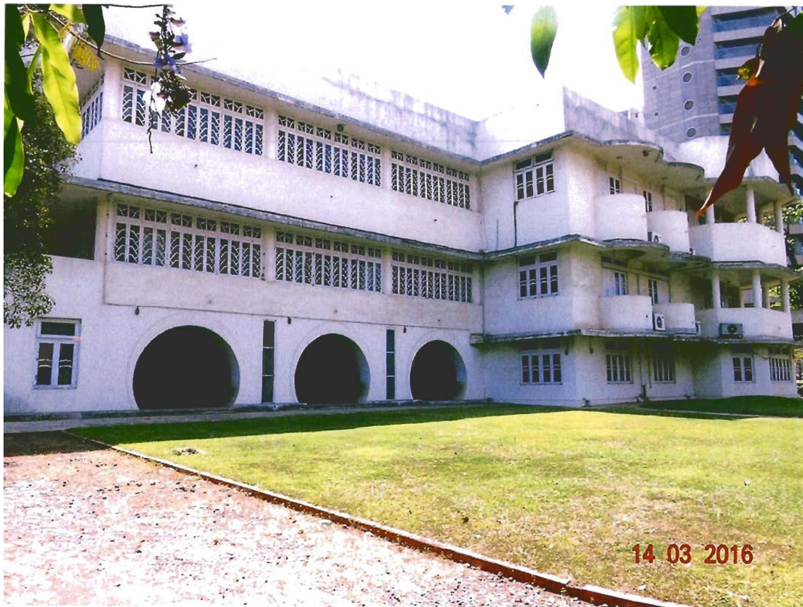
Figure 1.1: Photographs of Existing Buildings at Proposed Site
