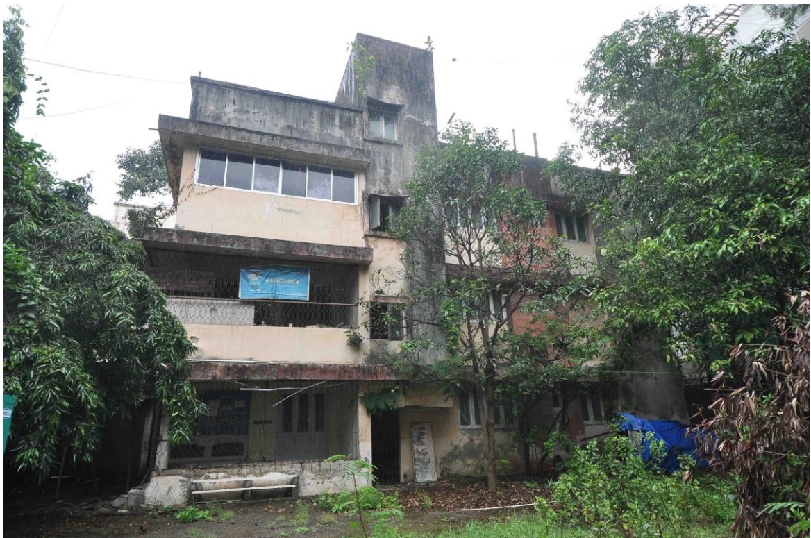
Figure 1.1: Photographs of Existing dilapidated Building at Proposed Site
