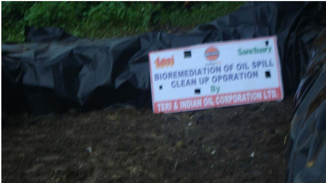
Pit after the completion of bioremediation.
