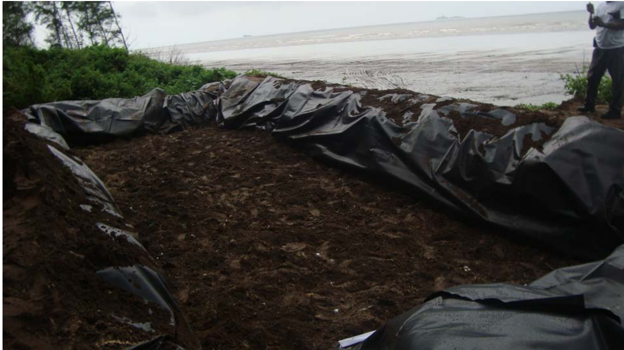
Pit after the completion of bioremediation.
