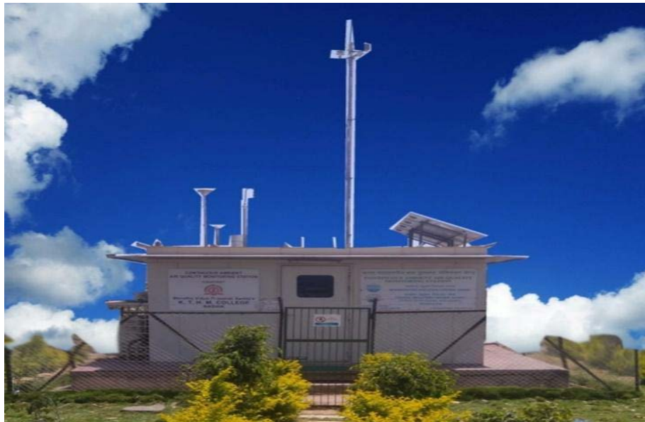
Continuous Ambient Air Quality Monitoring Station (CAAQMS)
