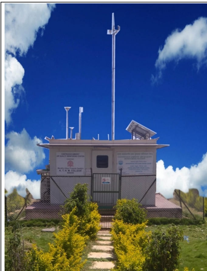
Continuous Ambient Air Quality Monitoring Station
