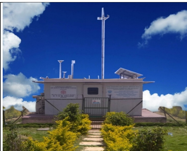
Continuous Ambient Air Quality Monitoring Station (CAAQMS)
