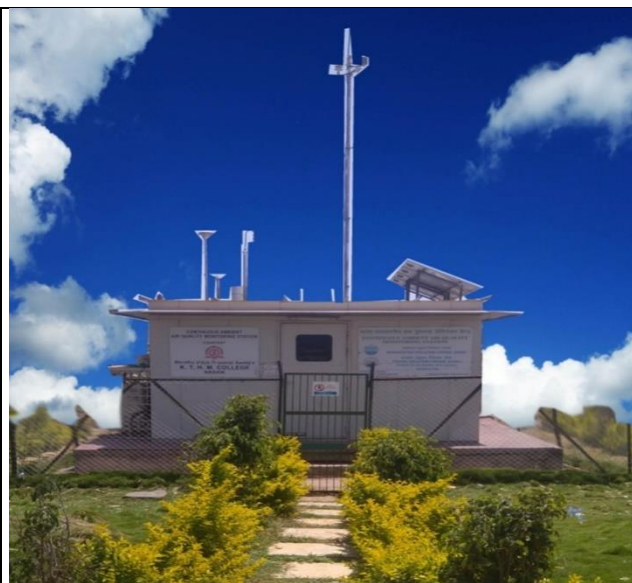
Continuous Ambient Air Quality Monitoring Station (CAAQMS)
