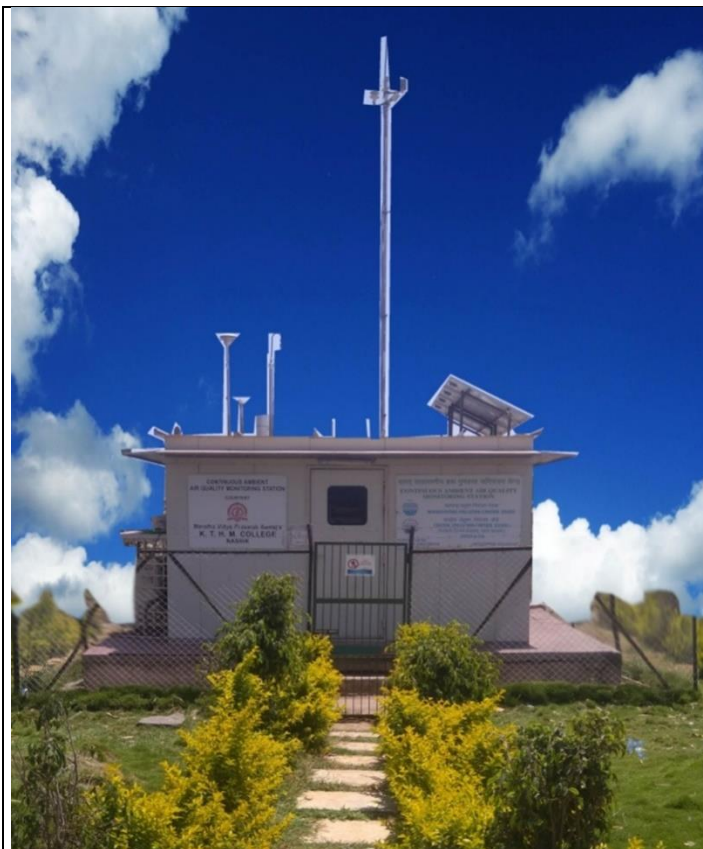
Continuous Ambient Air Quality Monitoring Station
