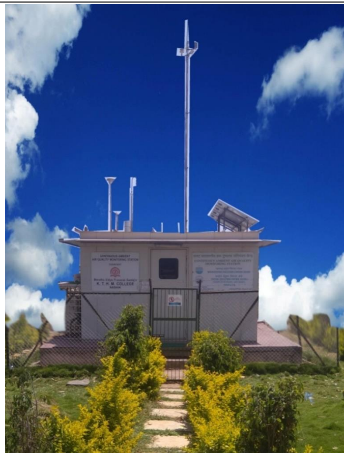
Continuous Ambient Air Quality Monitoring Station
