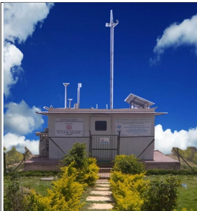
Continuous Ambient Air Quality Monitoring Station (CAAQMS)
