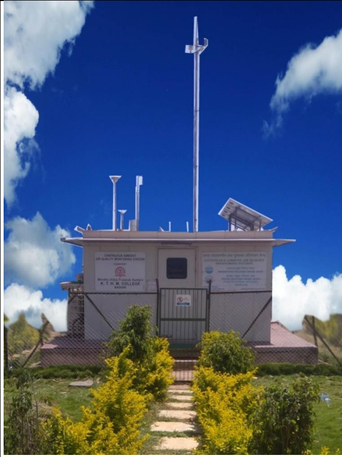
Continuous Ambient Air Quality Monitoring Station (CAAQMS)
