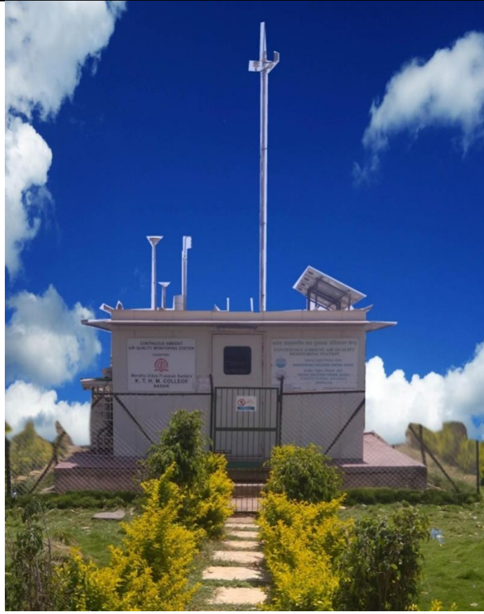
Continuous Ambient Air Quality Monitoring Station (CAAQMS)
