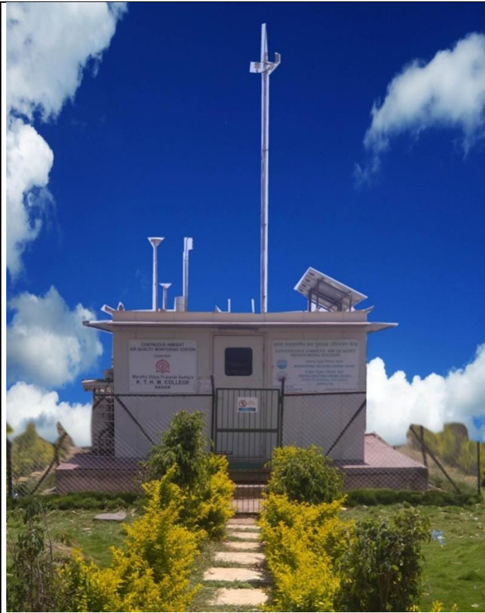
Continuous Ambient Air Quality Monitoring Station
