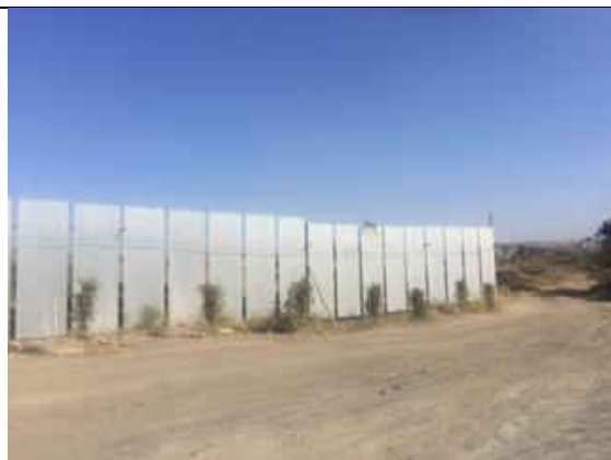
Photograph: the tin sheet barrier around the boundary which acts as wind breaking walls and small plantations
