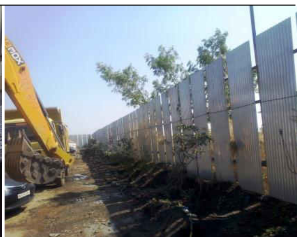
Wind breaking wall and plantation on the periphery for green belt development.
