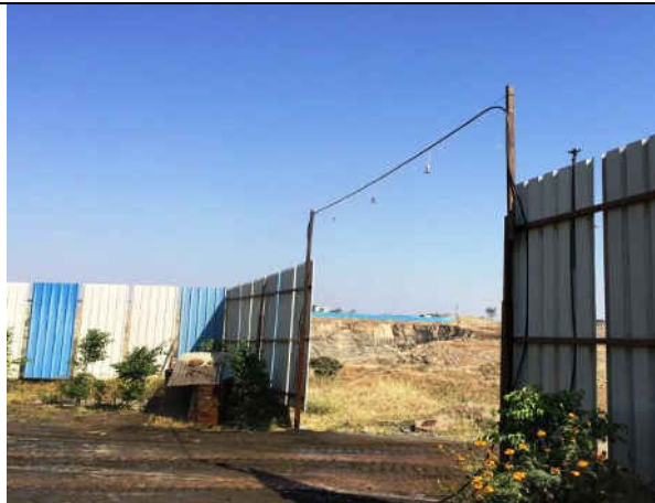
Fogger line at Entry and Exit gate
