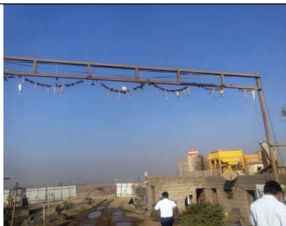
Overhead Foggers at Entry/Exit point.
