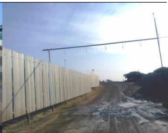
Overhead fogger provided at entry/exit point.
