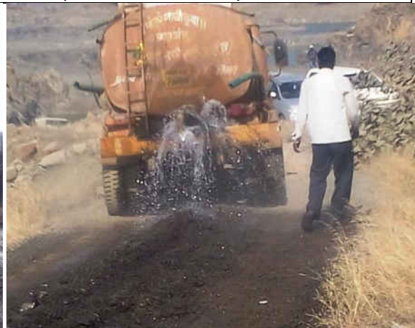
Excessive application of water through tankers inside the unit.
