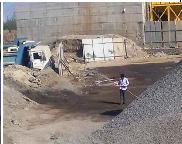
Ground wetting with flexible pipe.
