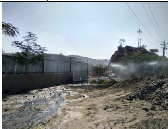
Photograph: Sprinkling system at the boundary
