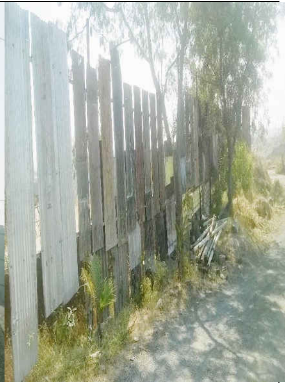
Photograph-2. View of a portion of wind breaking wall showing gaps between sheets.
