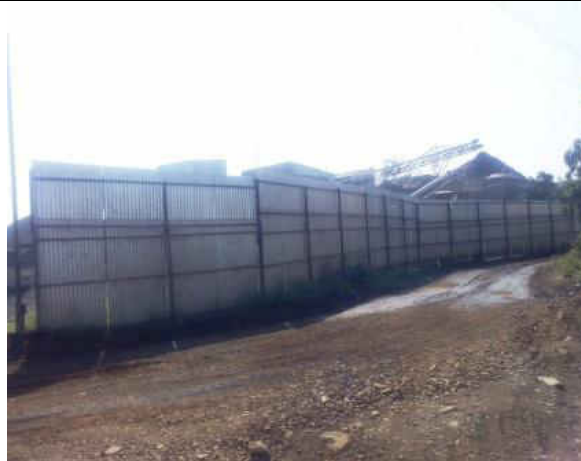
Height of material transfer point from conveyer is more than wind breaking wall.
