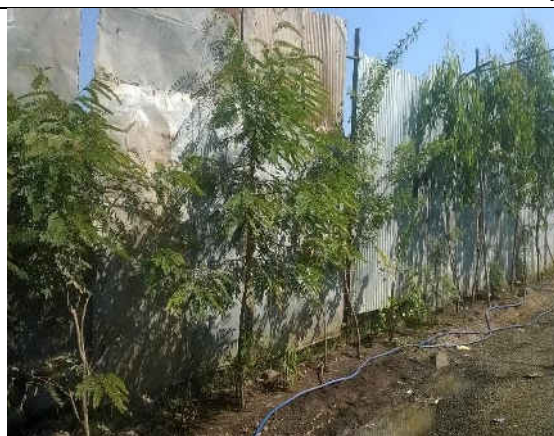
Photograph-2. View of a portion of wind breaking wall showing gaps between sheets and plantation.
