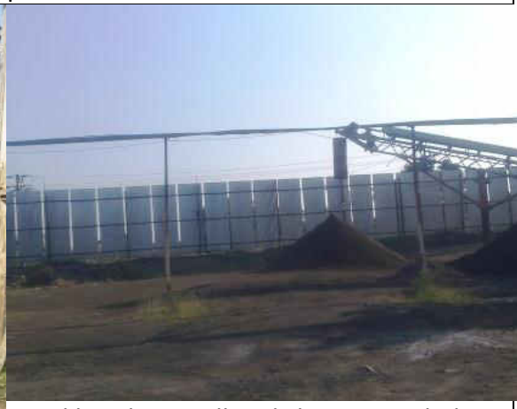
Wind breaking wall and chute provided to drop the material from conveyor at height lower than wind breaking wall.
