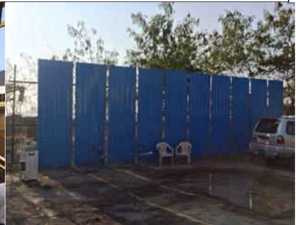
Wind breaking wall at one of the side of the unit
