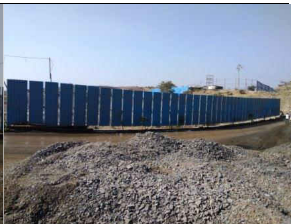
Photograph: Tin sheet barrier as boundary wall
