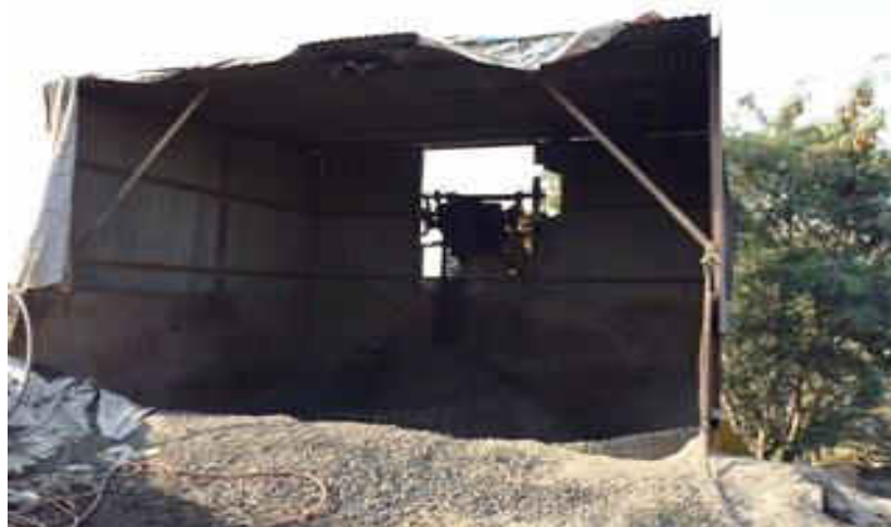
Hopper provided with tin shed from all sides except one kept for feeding through JCB or Poclain
