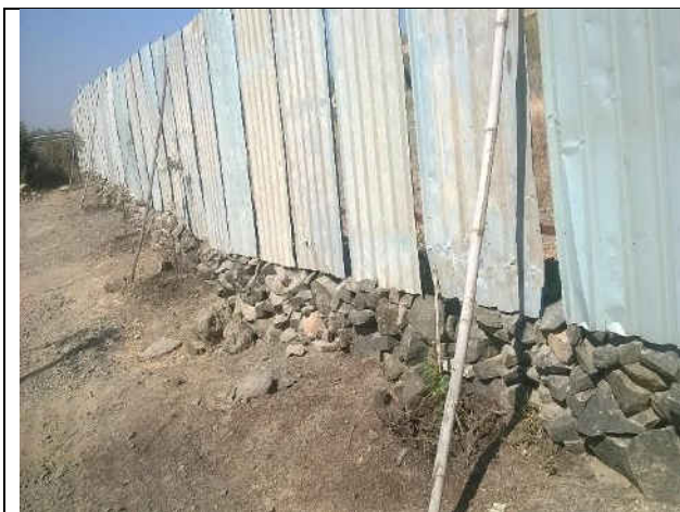
Photograph-1. WBW supported by bamboo column and one row new plantation at the spacing of 6-7 m.
