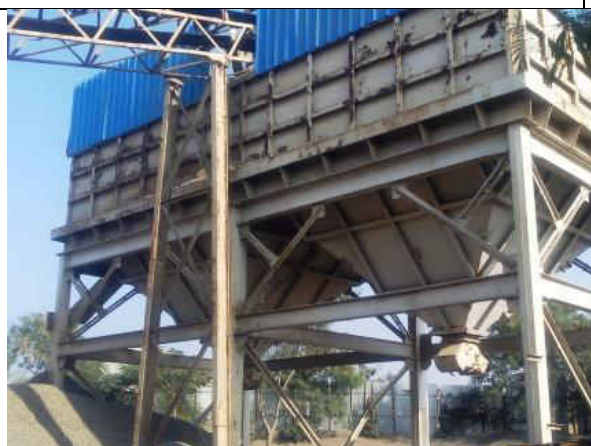
Hopper/Silos provided for product storage.
