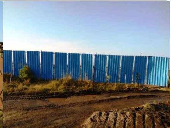
Photograph: tin sheet boundary wall with gaps
