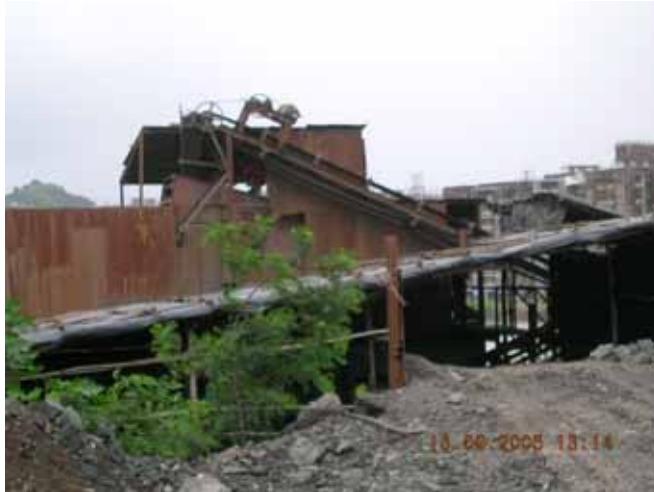
Photograph-3: M/s Supreme Stone Crusher in operation
