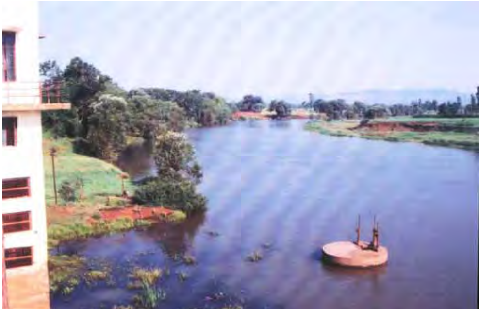
PANCHAGANGA RIVER - AT BALINGA WATER WORKS
