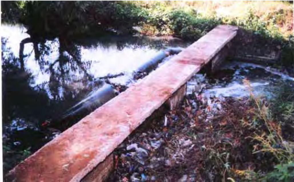
DUDHALI NALA - CARRYING SEWAGE TO PANCHAGANGA RIVER AT KOLHAPUR
