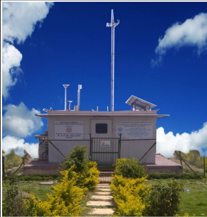
Continuous Ambient Air Quality Monitoring Station
