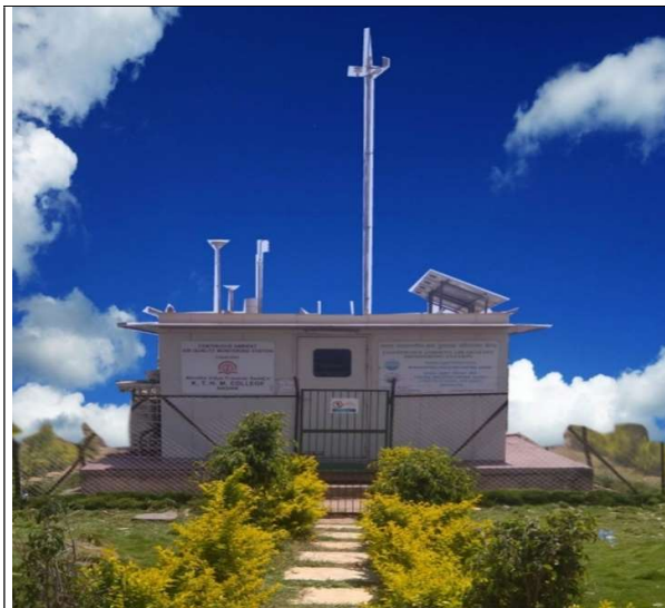
Continuous Ambient Air Quality Monitoring Station (CAAQMS)
