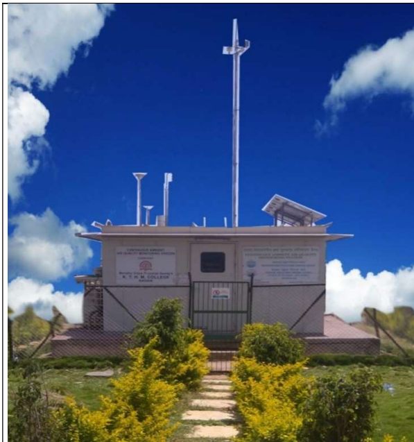
Continuous Ambient Air Quality Monitoring Station (CAAQMS)
