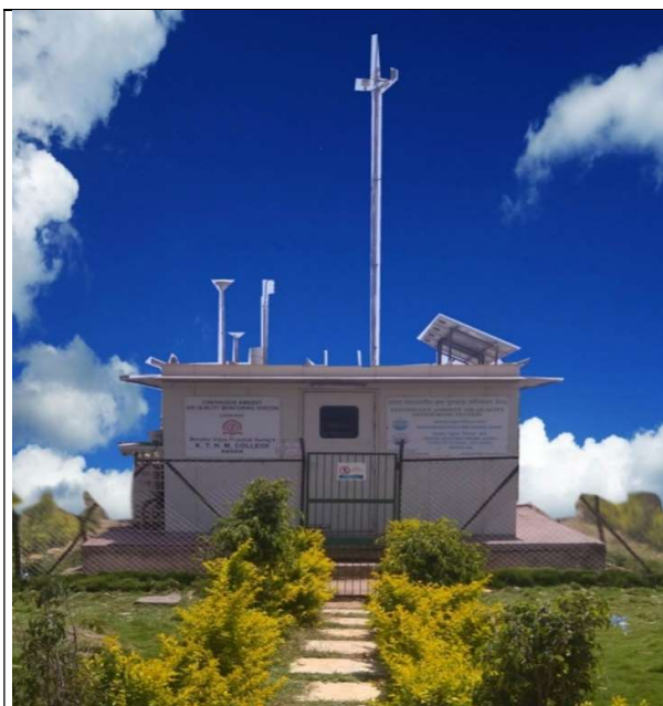
Continuous Ambient Air Quality Monitoring Station (CAAQMS)
