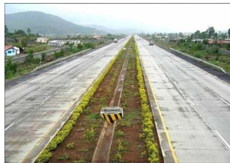
Plate 2. Mumbai - Pune Expressway
