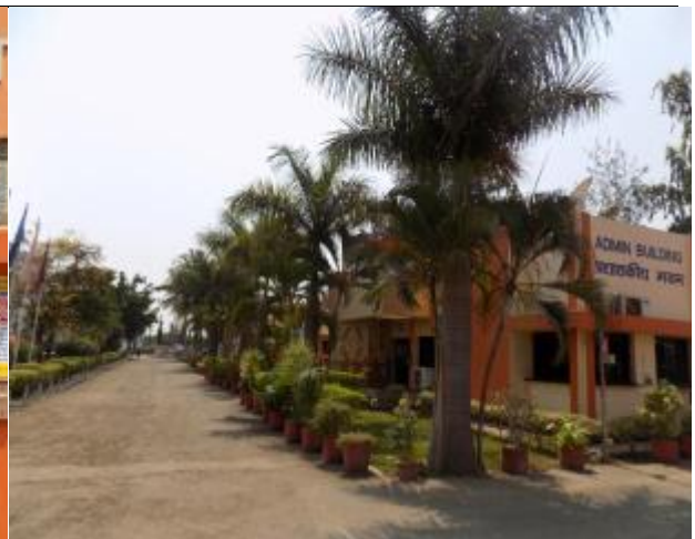
Admin Building Area
