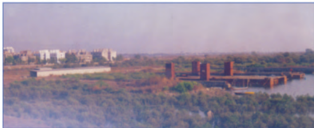
Fig. 10. The abandoned jetty & the other structures that were used for construction of Airoli bridge
