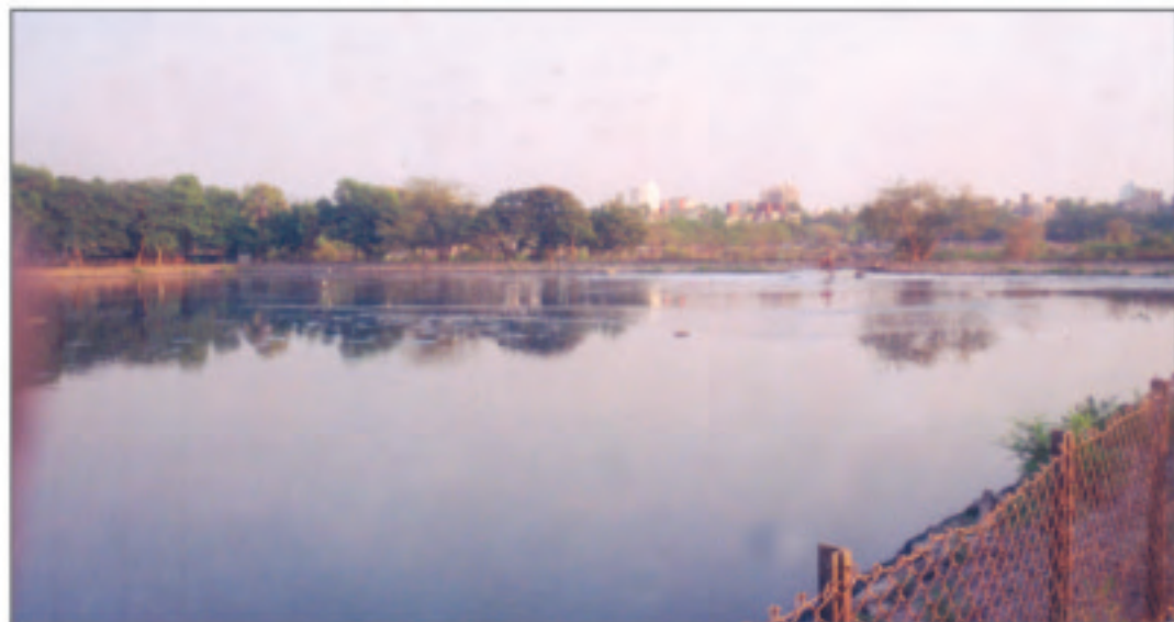
Fig. 2. Poorly maintained STP at Airoli
